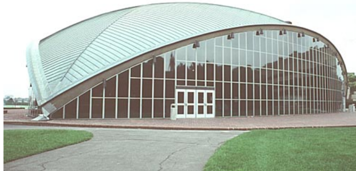
Figure 2: Roof shell constructed using reinforced concrete, Kresge Auditorium, MIT campus, USA [21].
